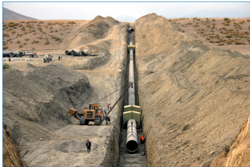
Construction works of Oguz-Qebele water pipeline
