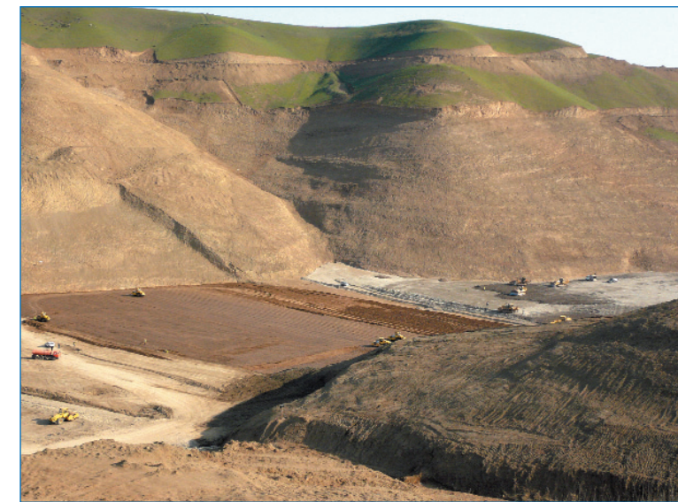
Dam building works in Takhtakorpu Water Reservoir
